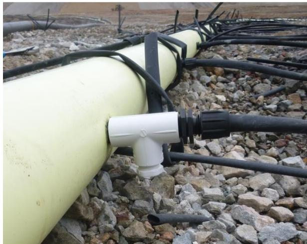
Figures 4 and 5: Design and Photo of EFV with Tee or Wye Fitting
