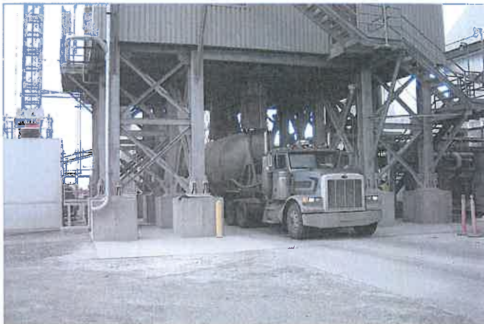
Figure 8 – Loading dry fly ash to bulk pneumatic trailer for transport and re-use offsite
