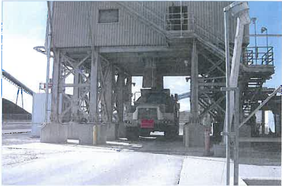
Figure 3 – Loading 20-ton TSPP Dump truck for transport of fly ash to landfill
